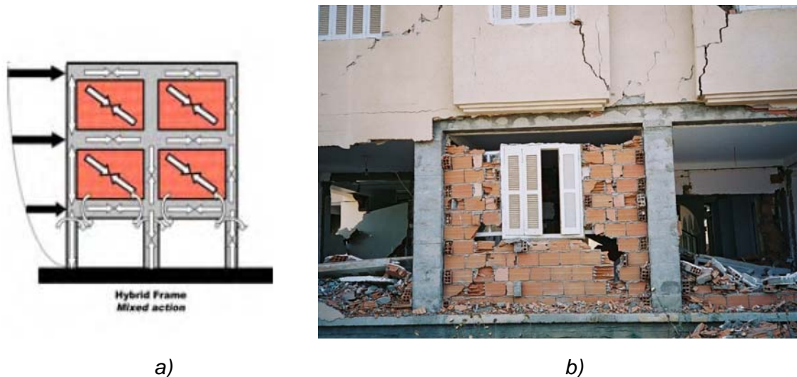
Figure 2-38. Soft storey mechanism: a) vertical discontinuity in masonry infills 2 ; b) building damage in the 2003 Boumerdes, Algeria earthquake 3 .
