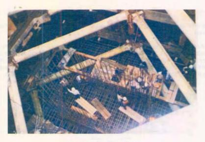
Fabrication of Steel Bar in Pile Cap
