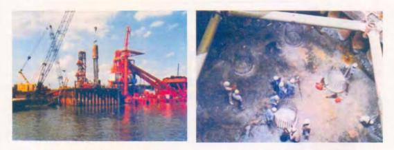
Insertion of Steel Bar Cage inside Bored Pile
