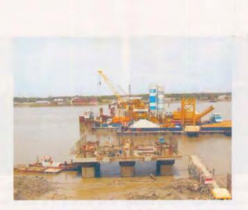
In order to construct pile cap below the water level the precast concrete shell forms were constructed and hanged around the steel casing for main piles above the water level
