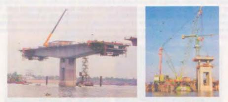
Balanced Cantilever Construction
