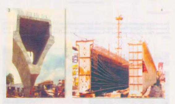
Y-frame Constructed in-situ for Supporting 44m Long PC Girders
