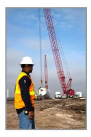
The biggest challenge on the Settlers Trail project was carrying out construction during the winter. Early spring delivery of the turbines meant that enough foundations had to be installed and backfilled so that trucks would be able to pull up to the foundation to drop off components for the cranes to pick up.
