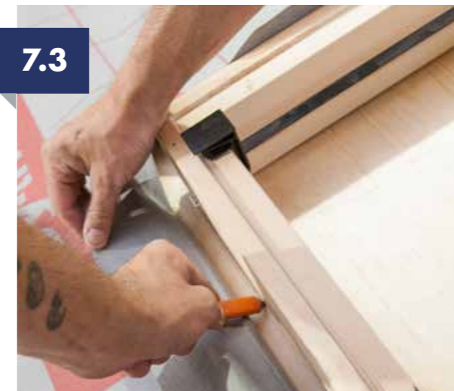
Reposition the frame and mark the position of the roof window on the plyboard.
