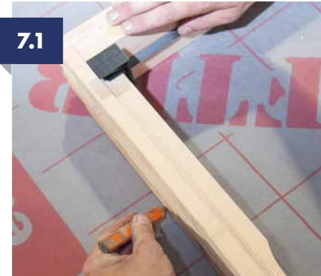
Before installing the roof window, install the first course of tiles. Place the roof window in position and mark the position of the roof.
