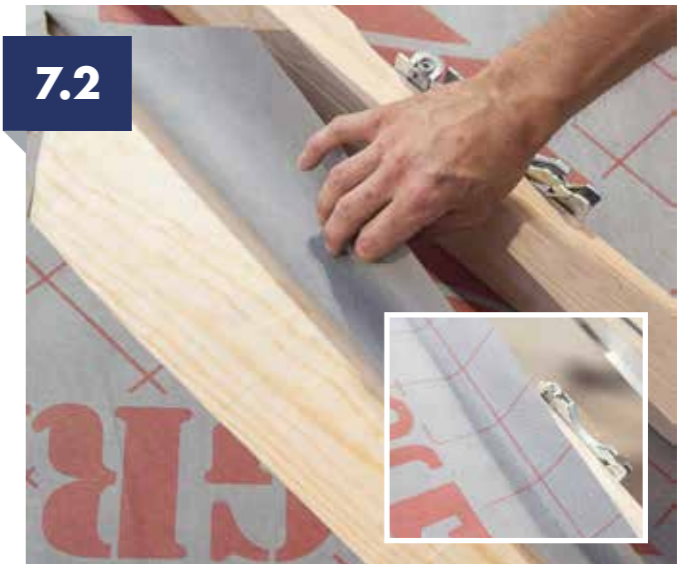
Cut the breathable membrane using a Stanley knife leaving at least 75mm on each side to overlap the outside of the frame (see inset).
