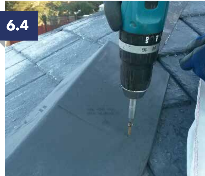
Affix ridge tiles using 2 x 30mm stainless steel screws.
