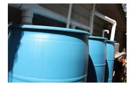
Water harvested from roofs and stored for irrigation
