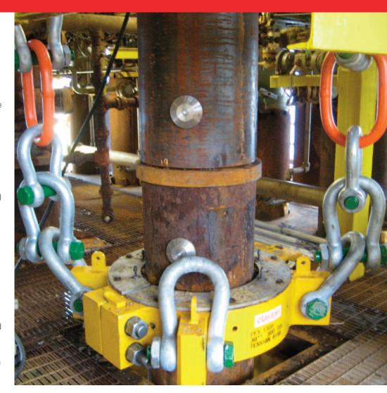
A Claxton tension ring securing a conductor during a recent slot recovery operation.
