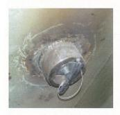
Permanently fitted Tube Socket. When build up occurs sealing plug is taken out and tube inserted through socket.
