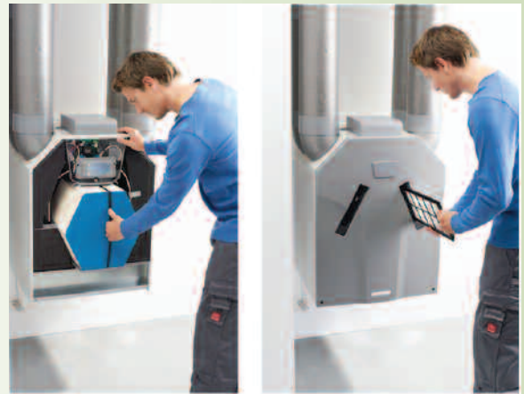
Cleaning the heat exchanger
