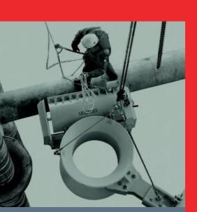
"TO HIGHLIGHT JUST SOME OF OUR EXPERIENCE IN THIS AREA: WE'VE INSTALLED MORE CONDUCTOR GUIDE CENTRALIZERS THAN ANYONE ELSE, MANY OF WHICH ARE RETROFIT DESIGNS, INSTALLED TO EXTEND THE WORKING LIFE OF CONDUCTORS ALREADY IN PLACE."
