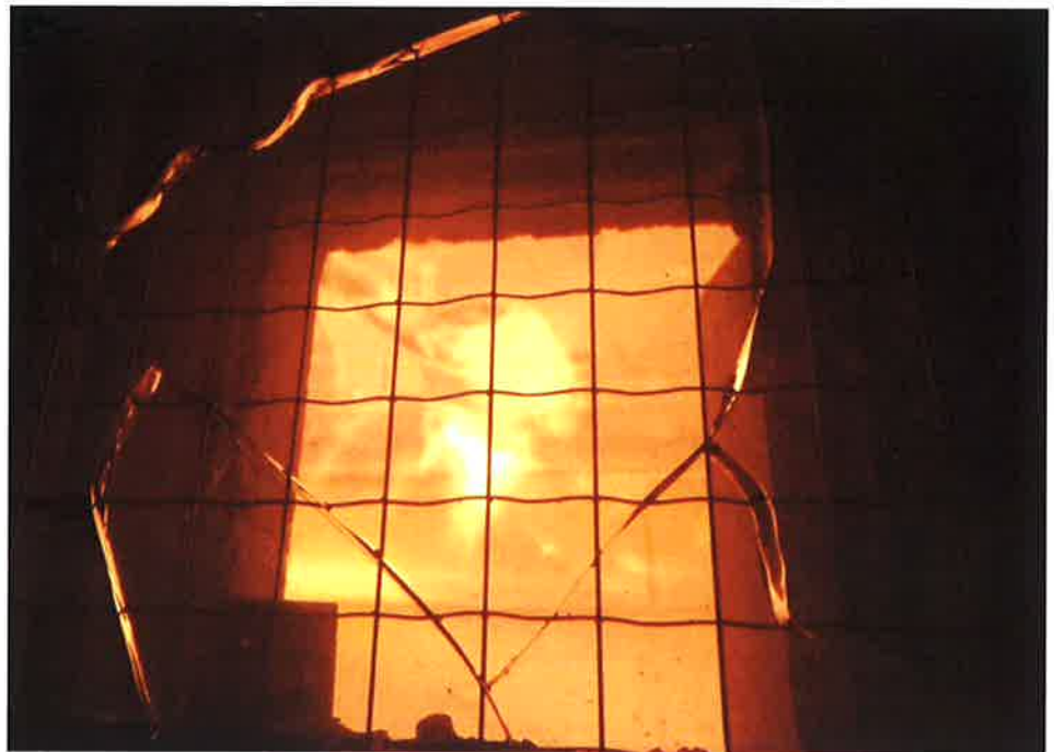
The exposed face of the ceiling after a test duration of 90 minutes
