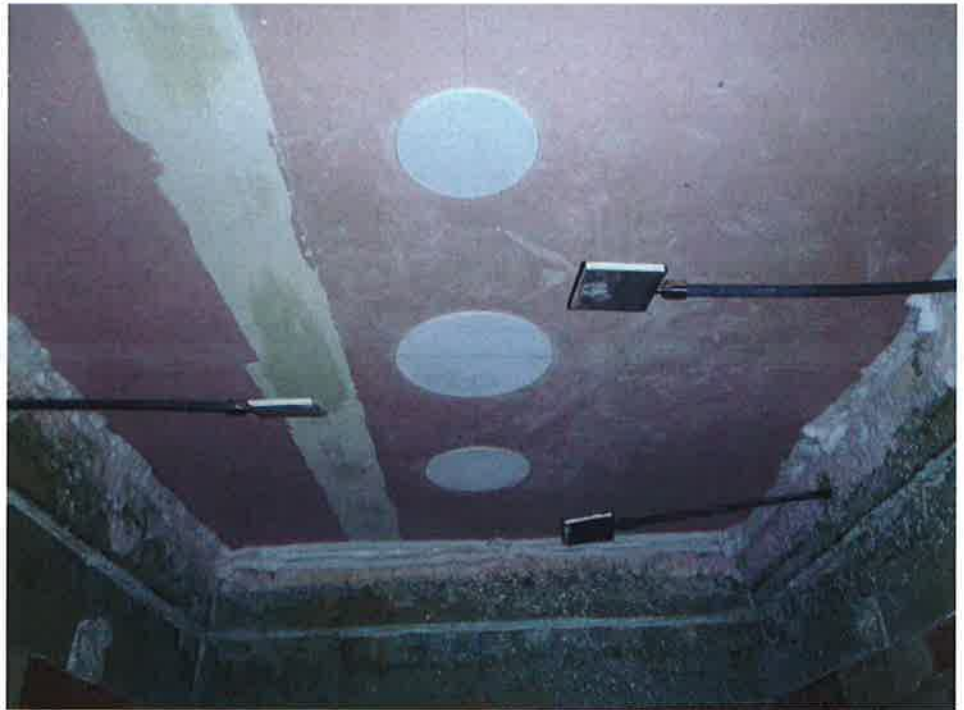
The exposed face of the ceiling prior to the test.
