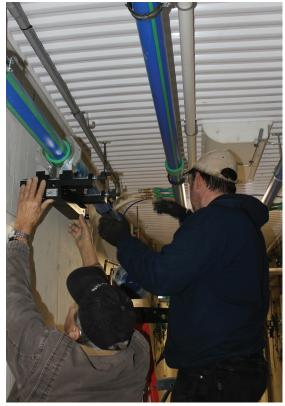
Technicians from Mid-Lam Heating & Cooling heatfusing Aquatherm pipe.
