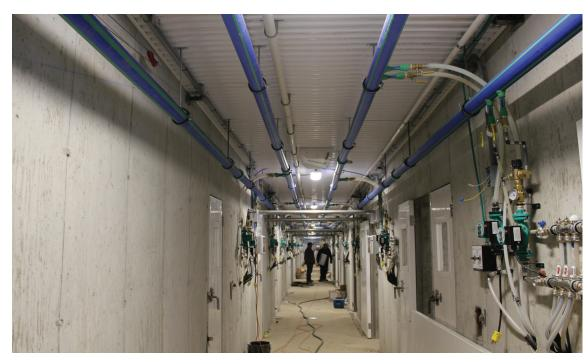
Aquatherm pipe during construction of this pig barn. The pipe's light weight and ease of handling made it easy to hang, and it now carries heated water to the four zones of this barn.
