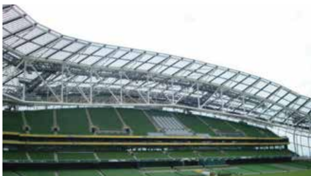
Aviva Stadium 18 Vandal resistant lifts, 51.700 spectators Dublin , Ireland
