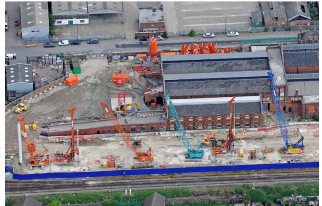
Crossrail Thames Tunnel C310 project
