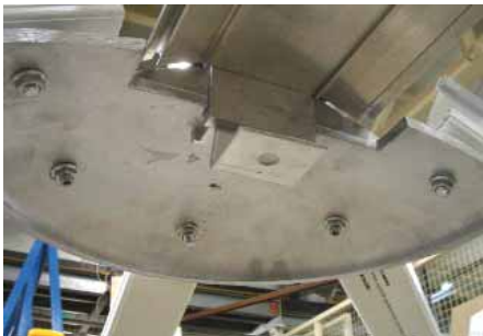
Picture showing the position of the tie-bar bracket once installed.
