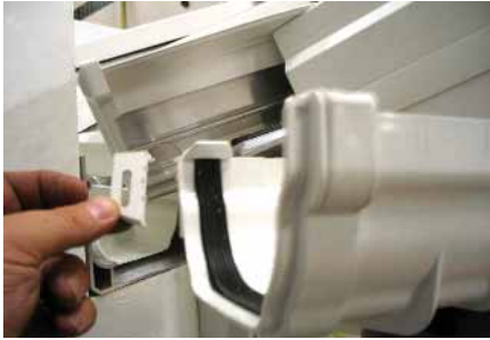
Remove the screw lug off the end of any gutter union that fits on to a box gutter adaptor.
