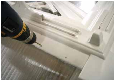
Position the ridge top cap corner cover XPT90 and drill 2 No. 5mm holes per side (8 total).
