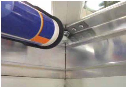
Eaves Beam: Seal all of the internal corner joints.
