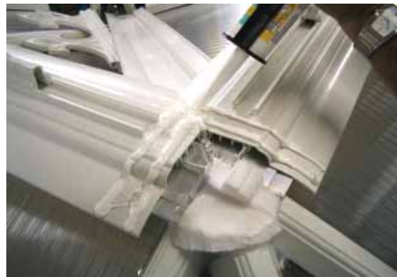
Apply silicone sealant to the ridge top in the area below the XPT90.
