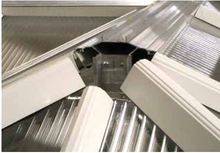
Fully glaze and cap all of the rafters, which fall onto the radius end.
