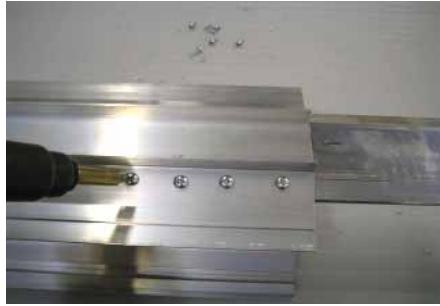
Secure the joiner with 4 No. XM48-13 screws each side of the ridge.
