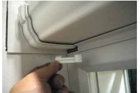
Finish off by fitting the main gutter and under gutter trims.
