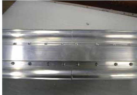
The view of the lower ridge joiner connected via 8 No. XM48-13 screws.
