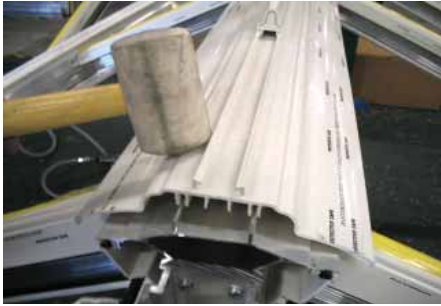
Centralise the two clips on the ridge top cap with the two bars on the main ridge.
