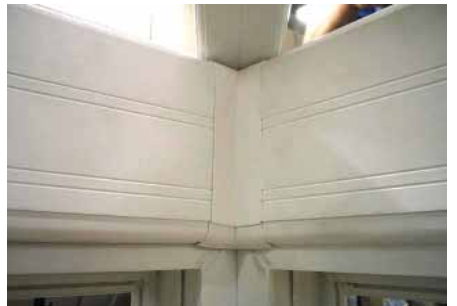
Slide the next section of eaves clad in to the eaves clad joint and knock the eaves clad in to position as before. Carry on with this procedure until all of the eaves clads are fitted.
