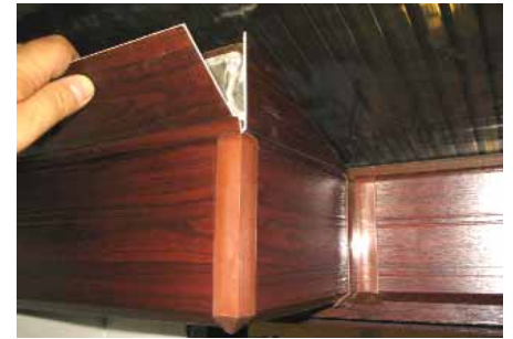
Measure and cut each individual section out of the extra under clad. This will clip down in to the already fitted side clad. The top will need to be fixed to the raised leg section with double sided tape or gunnable glue (not supplied).
