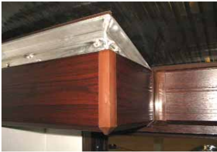
Raised Leg Box Gutter: Fit all of the internal side clads as standard.
