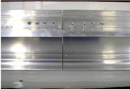
Slide the other ridge body onto the joiners and repeat the fixings procedure.
