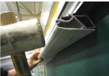
Wallplate Bottom Cap: Position the bottom cap making sure the bottom clip fits over the wallplates bottom barb. Using a rubber mallet knock the front bottom cap clip on to the wallplate in a continuous run from one end.
