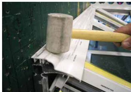
The PVC-U wallplate top cap is exactly half of a ridge top cap and is fastened in the same manner.
