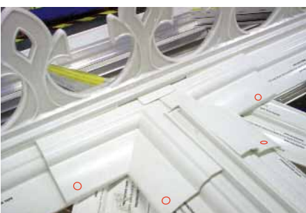
The run of crestings can now be slid along the ridge top cap over the joint. The bottom legs on the creasting should have been removed to allow this.
