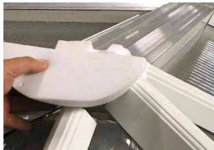
Test fit the half round foam bung making sure the chamfer runs downwards.
