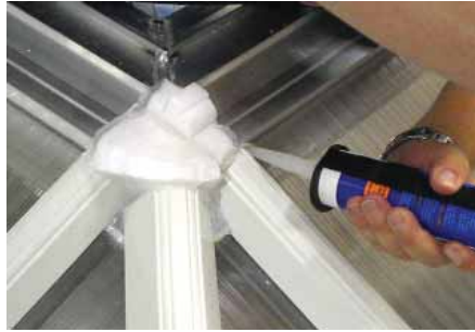
Completely seal the rafter top caps and roof sheets to the face of the foam bung. Seal the foam bung to the end profiles of the ridge.
