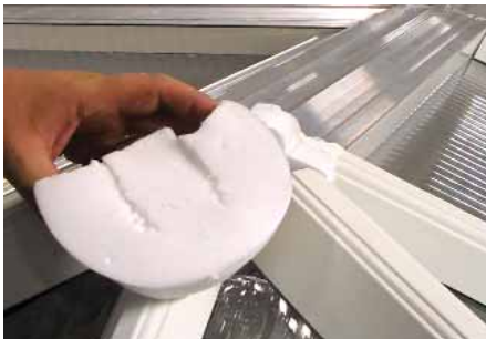
Adjust the size of the v-notches depending on the size of the aperture.
