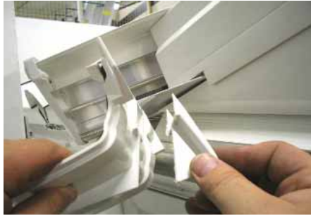
On straight unions the support webs will also need to be removed on the back and bottom sides.
