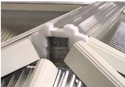
Insert the cut down section of bung making sure it is pushed firmly in to the silicone seal.
