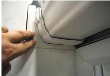
The end cap is then fitted by pushing it in to the end of the box gutter.
