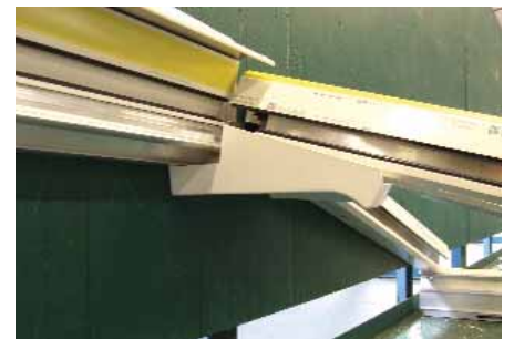
The internal half radius end cover should be scribed to fit around the wallplate.
