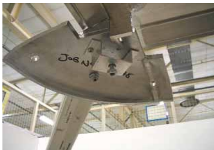
The internal half radius end cover is connected using the nut, bolt and bolt cap provided.
