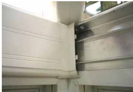
Place an internal eaves clad joint on to the end of an internal eaves clad. Position the clad over the eaves beam so that its clips line up with the eaves cladding barbs. Knock the cladding on using a rubber mallet.
