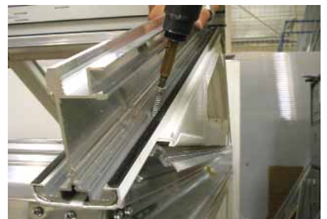
When a gable frame is used, the end rafter top and bottom bolts become redundant. Screw fix the end rafter to the head of the gable window as shown at 300mm centres.
