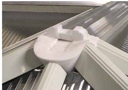
Push the bung in to the aperture so it finishes just above the rafter top caps.
