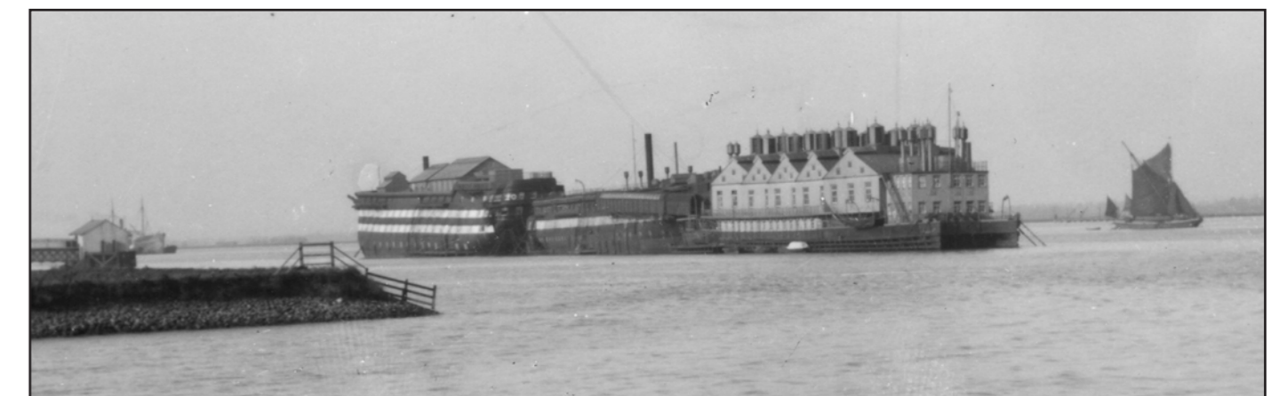
The hospital ships moored offshore at Long Reach - the Castalia is on the right.
