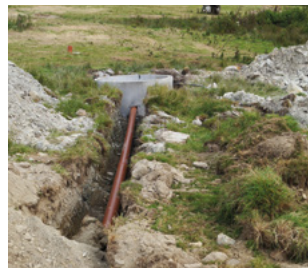
Installing the supply pipe from the supply tank to the pump chamber.
