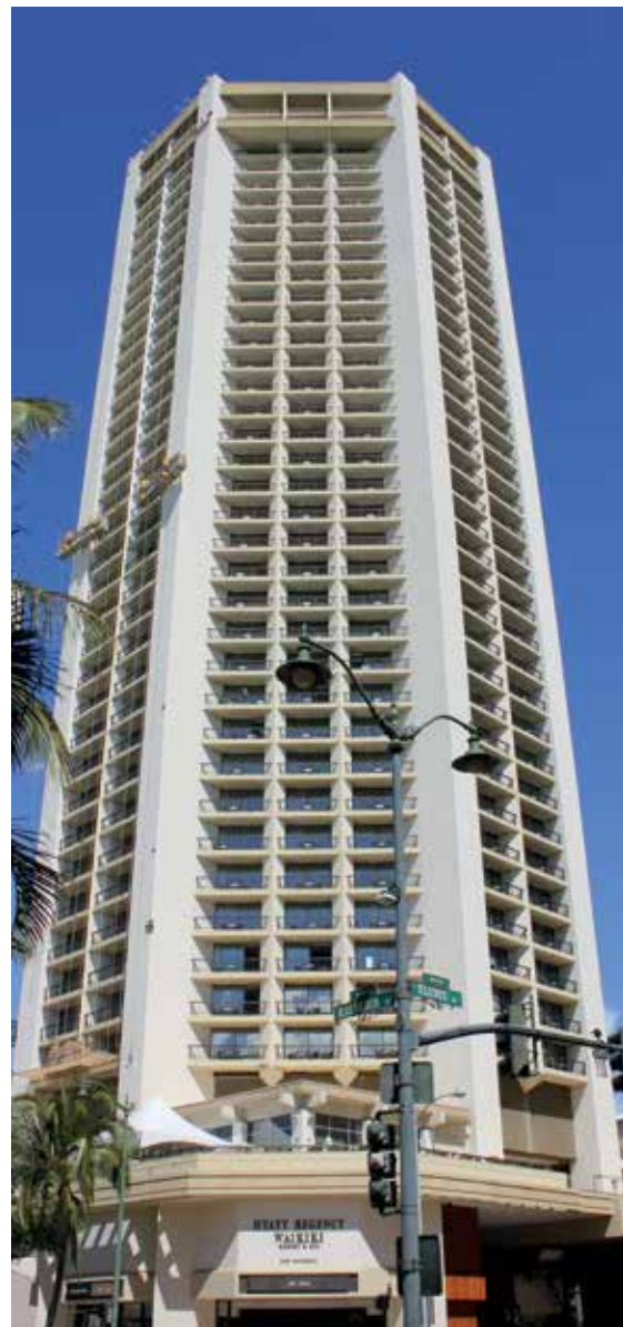
JD Painting & Decorating Inc. paints the Hyatt Regency. PHOTO COURTESY JD PAINTING & DECORATING INC.
