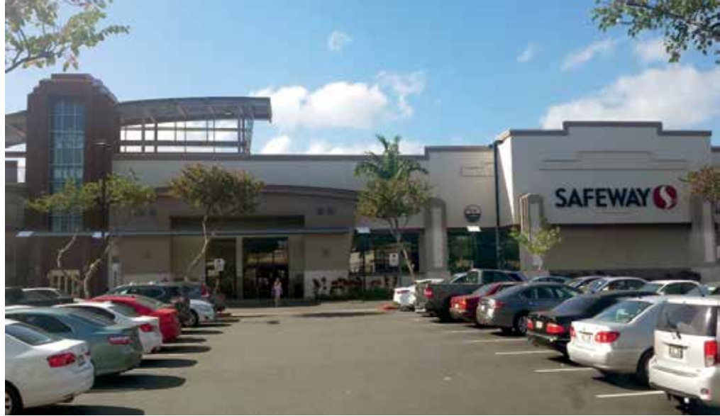
Kapahulu Shopping Center, a Benjamin Moore paint project PHOTO COURTESY BENJAMIN MOORE
