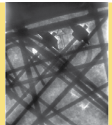
Slab with rebar, PT cables and anchors
