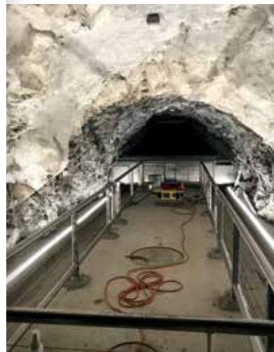
New stainless steel viewing window and railing with new accent pathway lights
