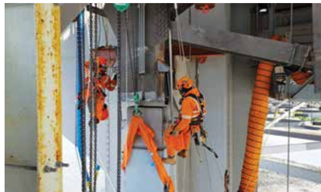
Replacement involved working in confined areas. Photo courtesy of Spencer Group.
