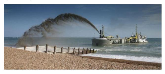
During the periods of **22<sup>nd</sup> – 28<sup>th</sup> January and 9<sup>th</sup> – 15<sup>th</sup> February 2020**, approximately 750m³ of shingle from the Owers Bank will be recharged to the beach around high tide to 1 hr after for approximately 14 high tides per cycle. Works will take place 24hrs, 7 days a week weather permitting.
