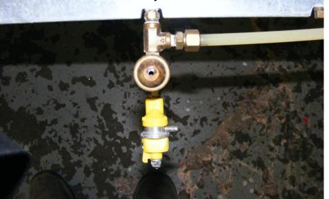
Plug off the supply inlet to the 3rd check valve for example
