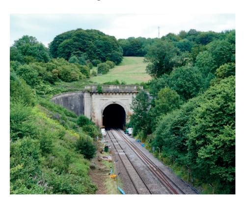
An impressive feat of engineering, Box Tunnel was dug from both ends and, when the two ends were joined in the middle, there was found to be less than 5 cm (or 2 inches) error in their alignment. Brunel had good reason to be proud of his accuracy.
