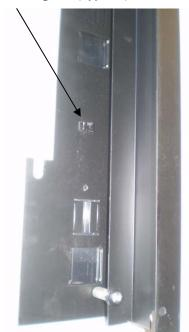
To remove the decorative trim from the glass rails it must be first raised upwards by approximately 5cm. & then pulled forwards.
