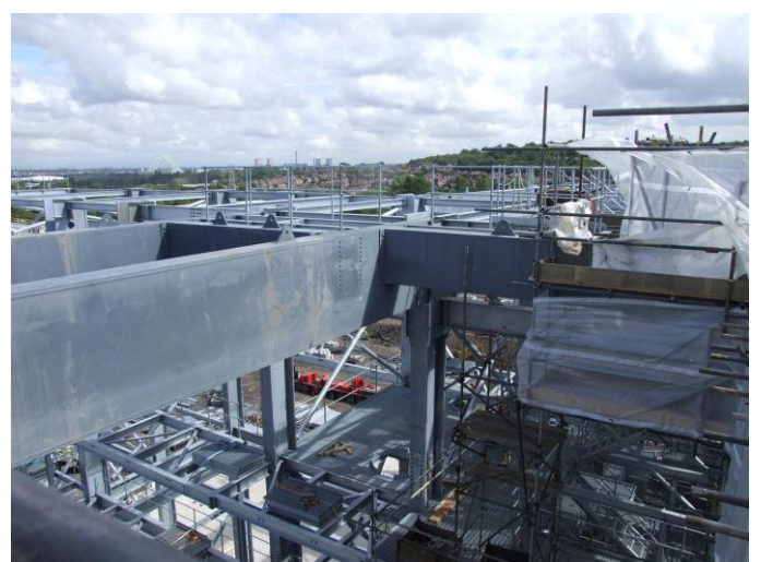
A view of the zingaised beams from above
