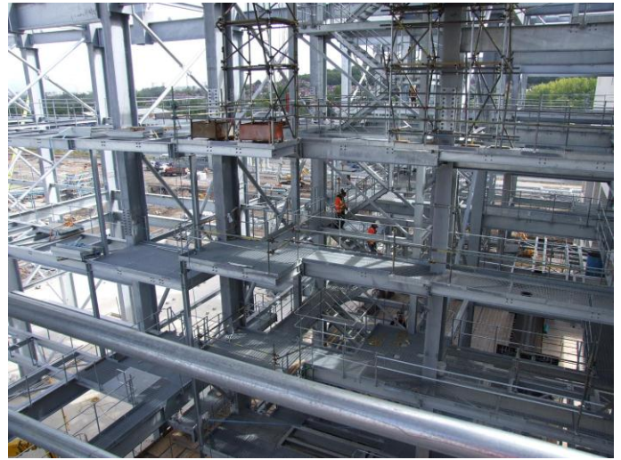
An aerial view of the steelwork showing the different levels
