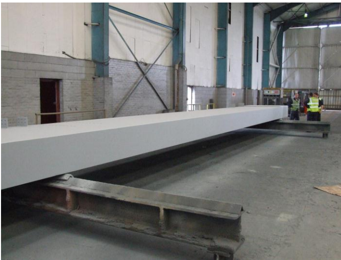
One of the 20-ton zingaised beams being checked
