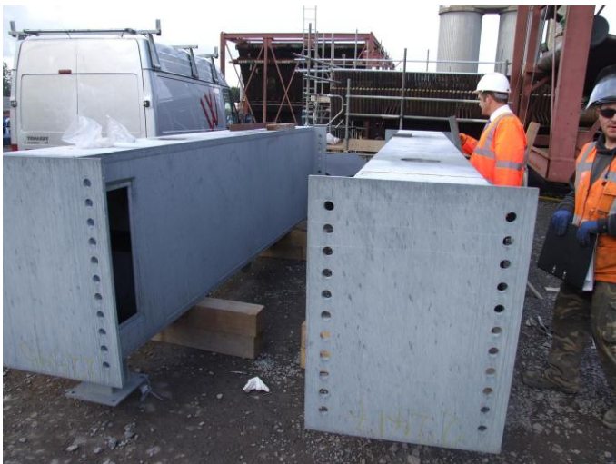
Checking the zinc-thickness on the zingansised beams
