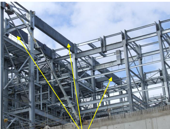
Zingaised beams in position
