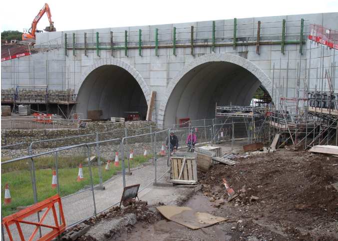
Camborne Pool Redruth East West Link Red River asset BEBO® Arches, asset VSoL Walls and Precast Containment Parapets all designed and supplied by asset International Structures Ltd.
