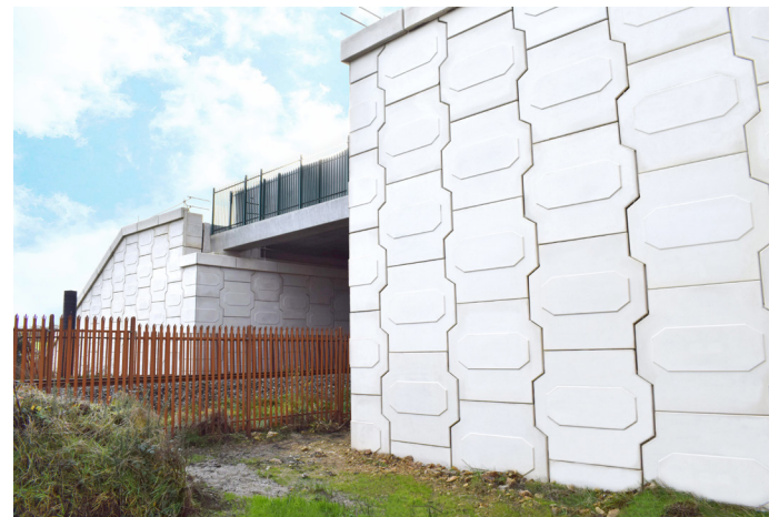
M11 Rail Bridge Scheme – asset International Structures Ltd asset VSoL Cross Panel.
