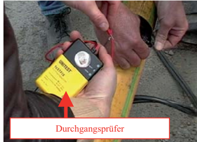
Fig 6-54: Verification of integrity using a continuity tester
