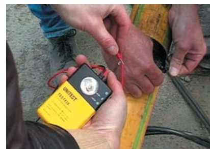
Fig 6-5: Verifying the integrity with a continuity tester
