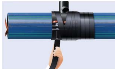
Fig 6-49: Wrapping the tapping fitting with Densolen Tape AS 40
