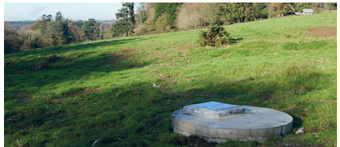
Water is captured high on the hill where there are natural springs.
