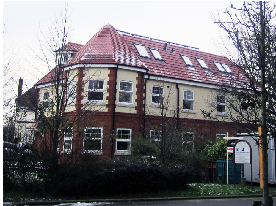
2 Avenue Road, Pinner
