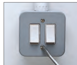
6 Fix face plate onto grid.
