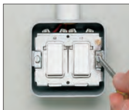
5 Fix wired switch/grid assembly into box.
