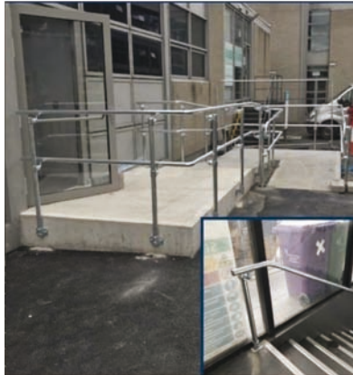
RTE DDA HANDRAIL INSTALLATION
