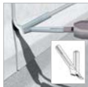
Perfect WR 41 wall weld
