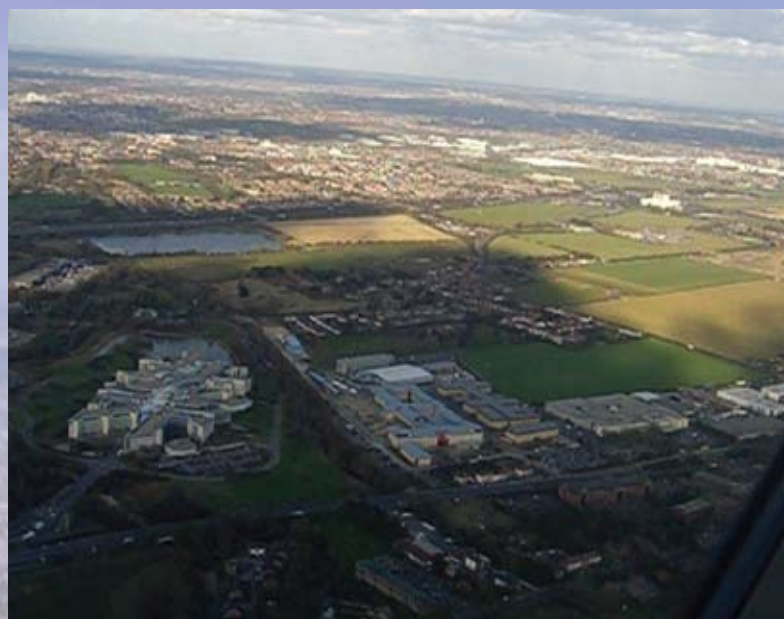
The site of the planned new third runway at Heathrow, with the BA Waterside Headquarters to the south west. (Editor's photo)
