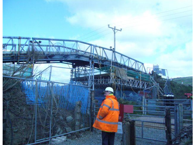
A view of the bridge during blast-cleaning operations
