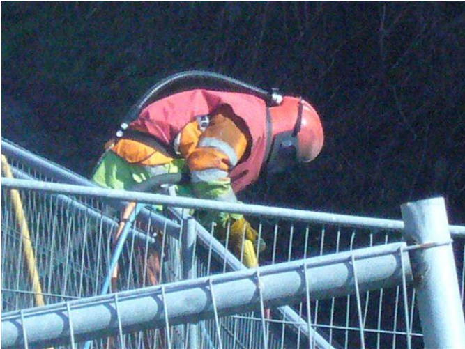
Blast-cleaning the bridge steelwork
