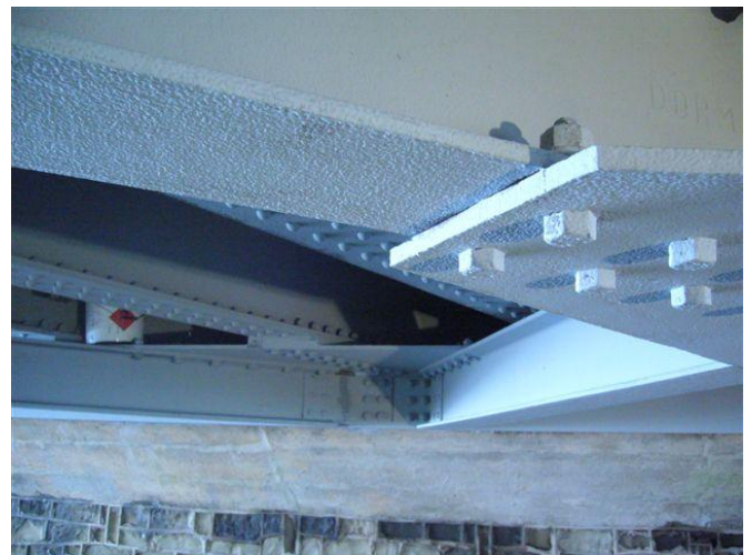
A view of some zingatised beams and fasteners
