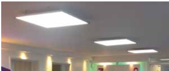
1200x300 Sigmalux LED Panel Suspended using mounting brackets
