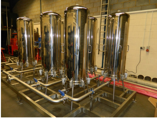
Skid unit and pipework assembly for client's filters
