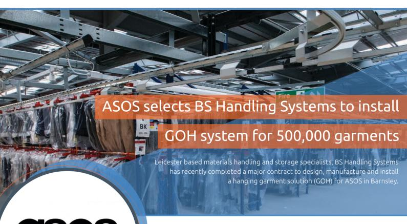
The innovative system includes a 30m long ladder conveyor to transport garments up to a 10m high mezzanine, GOH racking for half a million garments, a Slickrail system to move items into and out of store locations and a decline conveyor to automatically transport them back down to the 6m mezzanine level for packing.
