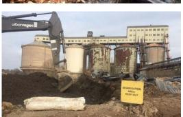
Post award of the main contract to Urban Regen Ltd., targeted instrusive investigation at the location identified significant volumes of heavily contaminated, heavy end TPH and associated PAH, both within and around the former structure.
