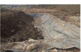
A temporary treatment area was prepared on an area of hardstanding, lined with dual gauge visqueen. As part of the overall strategy, water monitoring points were established to assess the risk to groundwater and subsequently the adjacent water course. This was supplemented with monthly surface water monitoring.
