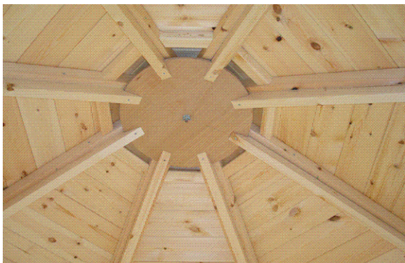
INTERNAL ROOF FINISH ON OCTAGONAL BUILDINGS
