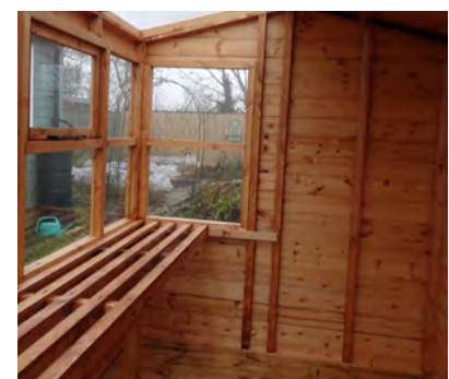
INTERNAL VIEW 1/2 GLASS ROOF & BENCH
