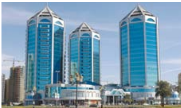
Crystal Plaza Towers in Sharjah, United Arab Emirates
