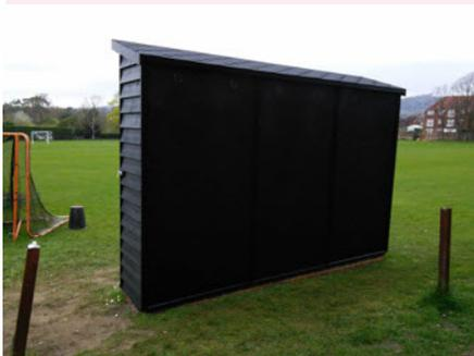
With the wiring complete and the board tested, signboards and the three back panels were fitted. Removable wooden shutters were installed to the front of the scoreboard for added protection.
