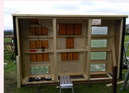
Once the front and side panels had been fitted the LED digits were installed whilst the roof was fitted and covered with shingles.
