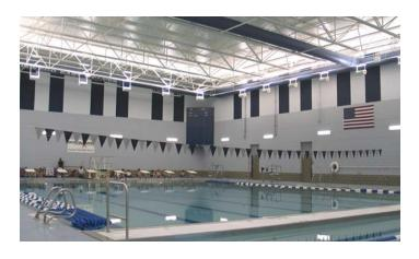
has a perimeter air distribution system of custom blue, 26-inch diameter fabric duct supplied by a 33,000-cfm Des Champs Laboratories, Natural Bridge Station, Va., combination dehumidifier and air-to-air heat exchanger. The duct is hung with corrosion-proof #316 stainless steel cable drops. Water Technologies, Milwaukee, Wis., was the natatorium consultant.
