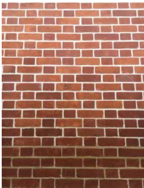
Hastings Medium Red and Dark Red built with lime mortar.
