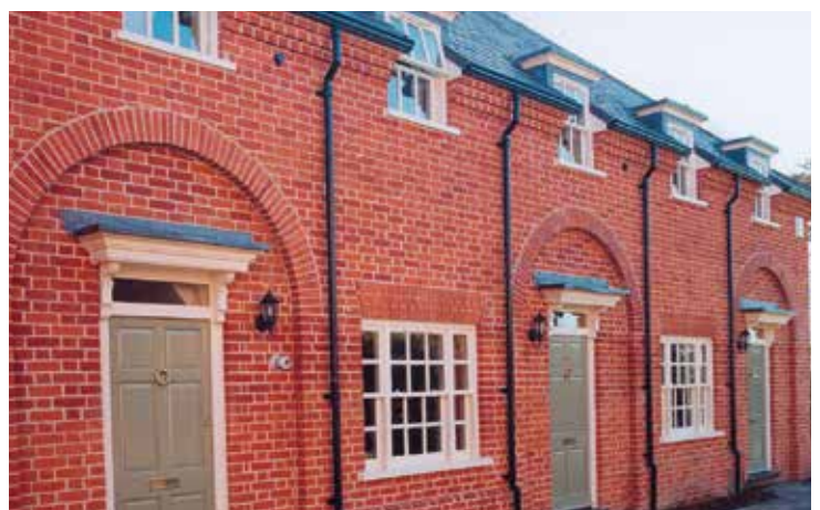
Russell's House built using a blend of Guestling Red and Waverley Orange bricks.
