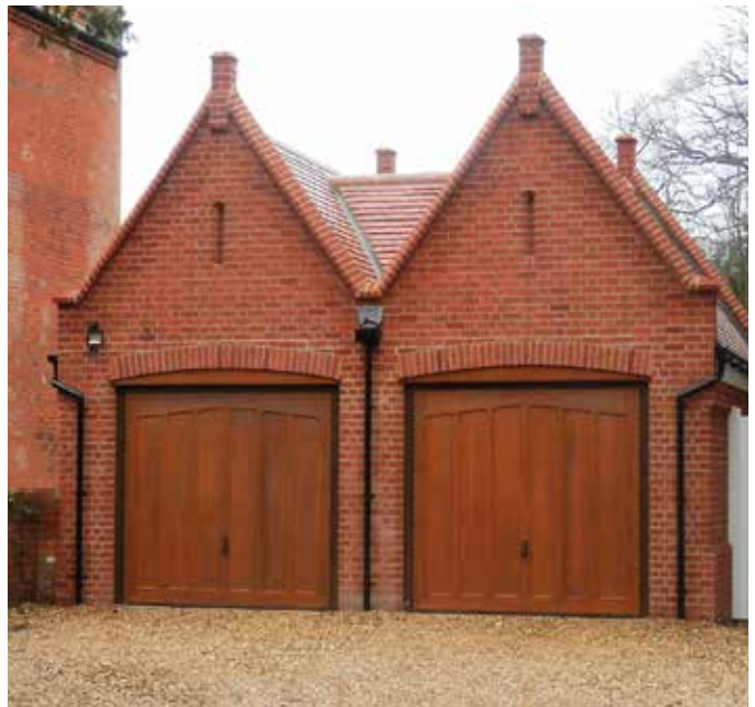
Private property in Ipswich built using a blend of Henley Red, Guestling Red and Westfield bricks.
