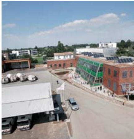
Municipal sanitation. Hamburg's municipal sanitation services reuse the water from showers and basins to clean the city.
