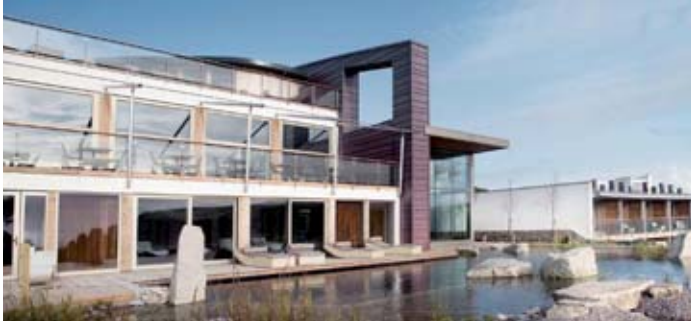
Scarlet Hotel, Cornwall. Hansgrohe products: Raindance overhead shower, Talis S basin mixer and Pontos AquaCycle 9000.
