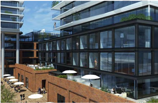
Figure 3.35 Podiums (brick and black portion of example) and towers setbacks should be used to create a pedestrian scale at grade (Distillery District, Toronto)
