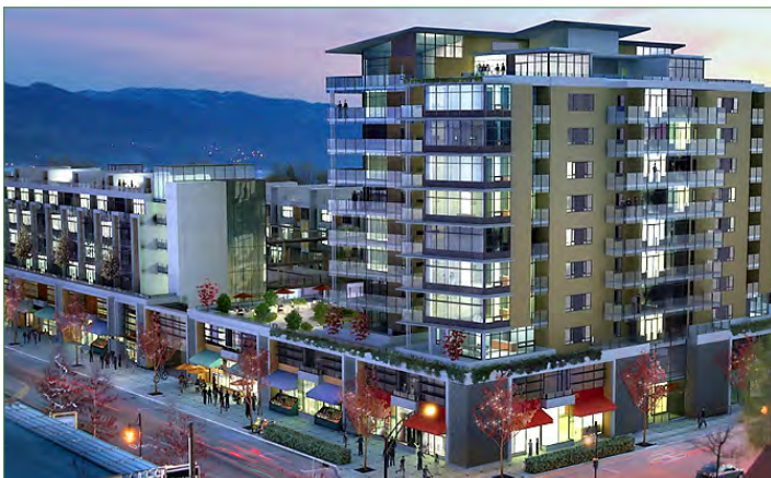
Figure 5.13 Continuity of the podium produces a transition for the difference between mid-block buildings and the gateways in the corners (SOPA Square, Kelowna BC)
