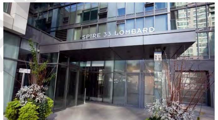
Figure 3.6 Canopies are required to protect building entrances from rain and wind (The Spire, Toronto).
