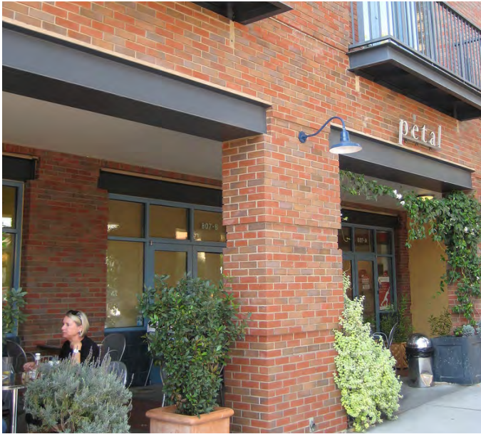
Figure 5.10 A setback at grade level can create a welcoming semi-open space for retail activity as well as weather protection
