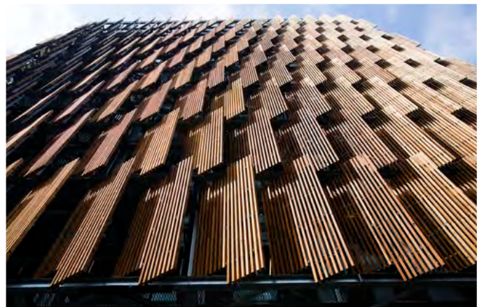
Figure 3.42 Innovative solar shades can control the amount of natural light that enters the building.
