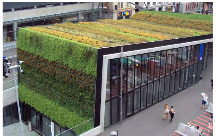
Figure 3.33 Landmark buildings should incorporate raised gardens and green-roofs, (ideally) accessible to the public (Flon Station, Switzerland)
