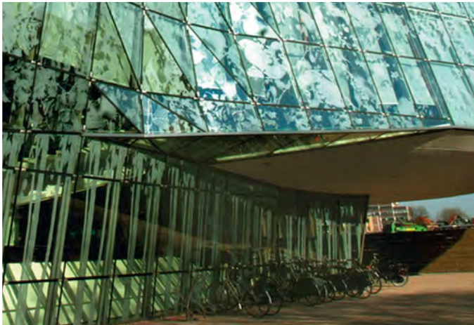
Figure 3.43 Articulation or treatment applied to glass project enough visual markers to make it visible to birds
