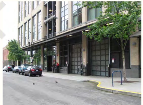
Figure 5.16 Access to servicing, loading and parking treated as a part of general architectural wall design.
