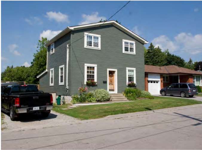
Figure 7.2 Existing Detached Home
