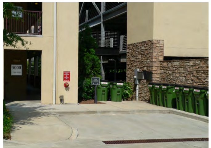
Figure 3.22 Centralized garbage rooms save space and help to minimize the impact of garbage collection services.
