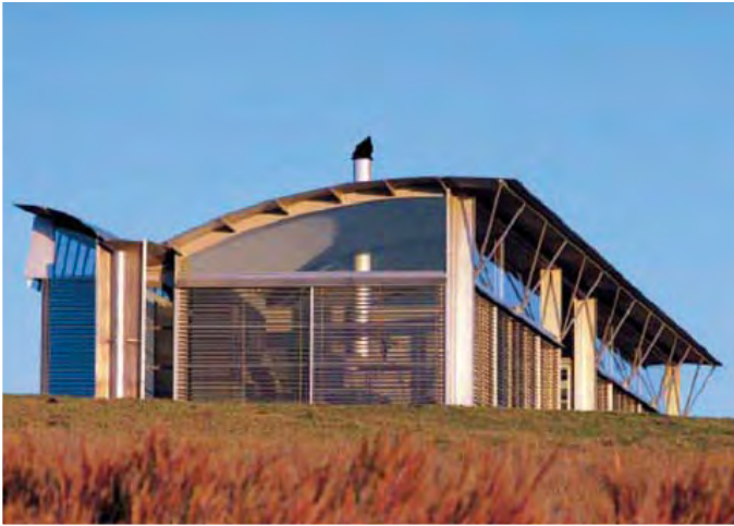
Figure 3.38 Roof design can help to collect and funnel rain water (Glen Murcutt's house, South Wales)
