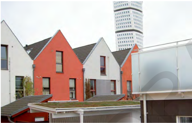
Figure 3.50 Green roofs can be also incorporated in lighter structures such as garages (Malmo, Sweden)
