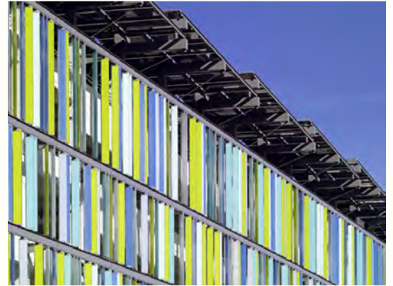
Figure 5.15 Parking structure walls should be concealed from the public realm by means of architectural treatment or screening (Santa Monica Civic Center Parking Structure, LA)
