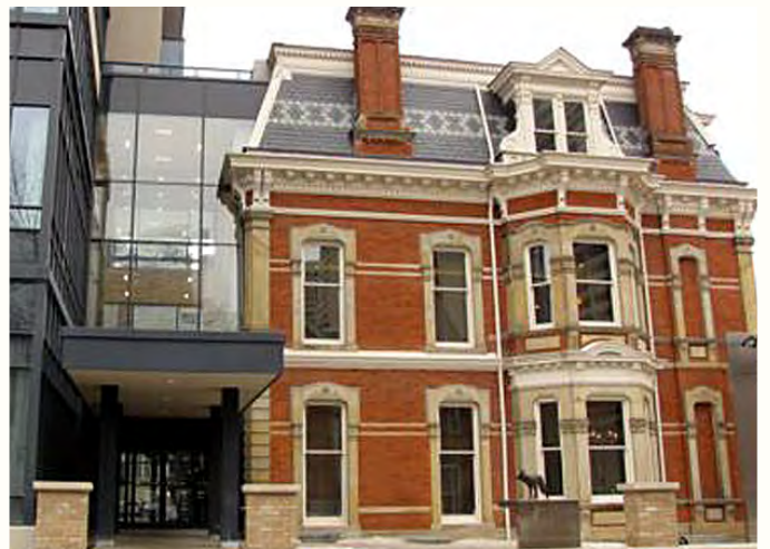
Figure 5.21 Renovation of buildings of historical significance should be made with attention to matching existing materials and historical architectural language, new construction should distinguish itself from historical components.
