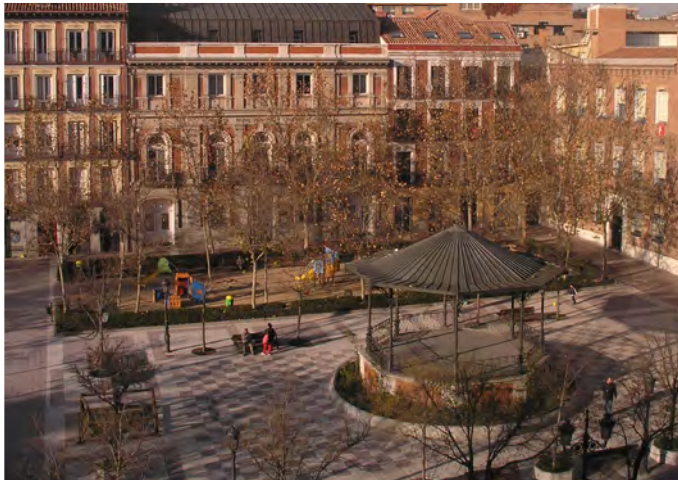
Figure 3.14 Deciduous trees allow the sun to access the streets and squares in winter
