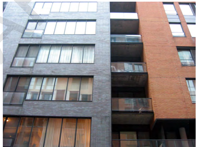
Figure 3.12 Brick façades are high quality and durable
