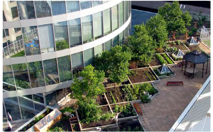
Figure 3.46 Rooftop gardens can be a source of local food (YWCA Vancouver, photo by Michael Levenson)
