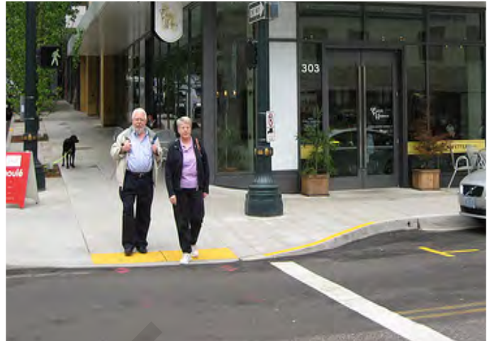
Figure 3.36 Well designed curb cut and markings ensure road safety and accessibility at the public realm.
