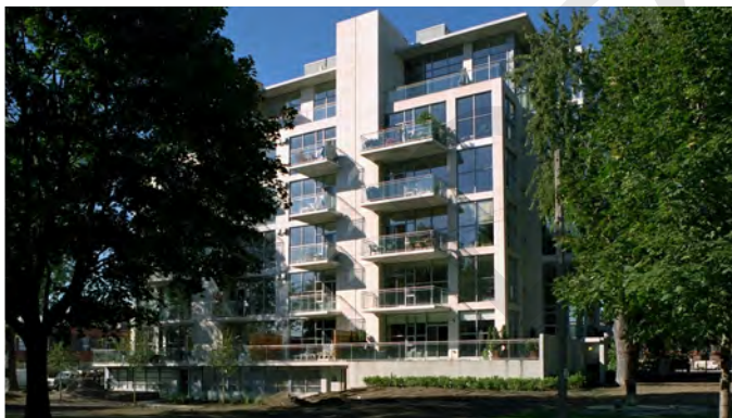
Figure 3.4 Balconies extend private outdoor space and create a direct connection with other landscape amenities (20 Niagara, Toronto)
