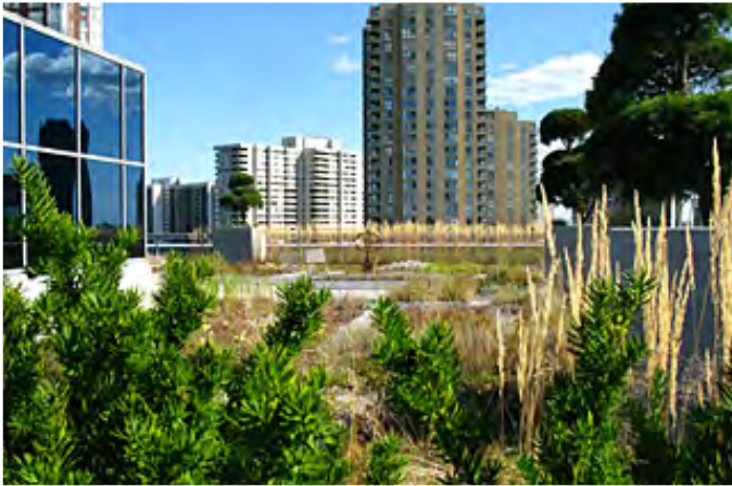
Figure 3.49 Green roofs reduce storm water run-off (Sears Merchandise Lofts Building, Toronto)
