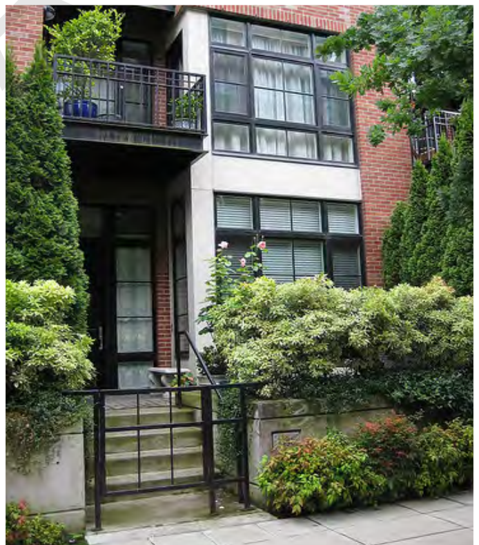
Figure 3.2 Entrances to townhouses may be elevated up to 1.5 m above grade and should be well defined
