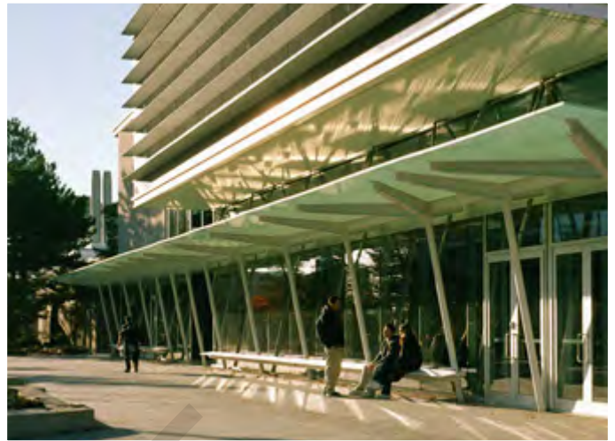
Figure 3.5 Canopies and awnings provide weather protection and help give a human scale to buildings
