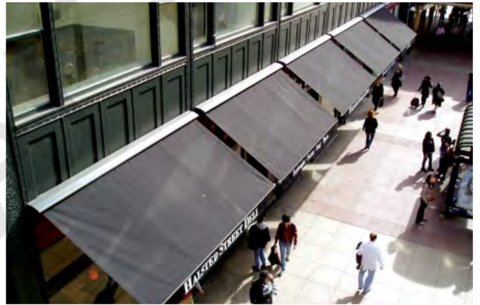
Figure 3.41 Operable shading has the benefit of providing shade in summer and allowing solar access in winter.
