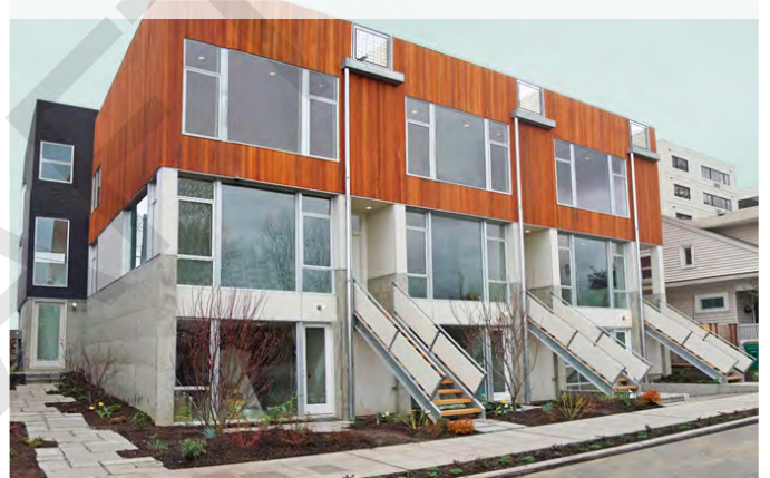
Figure 3.27 Buildings should face the streets while parking should be consolidated in the back, minimizing the number of driveways and access points to laneways
