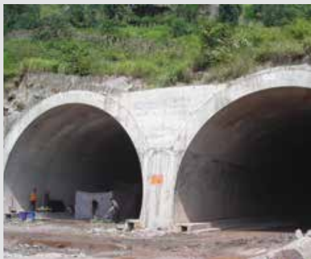
Repair work on the Yunnan Shuima Tunnels
