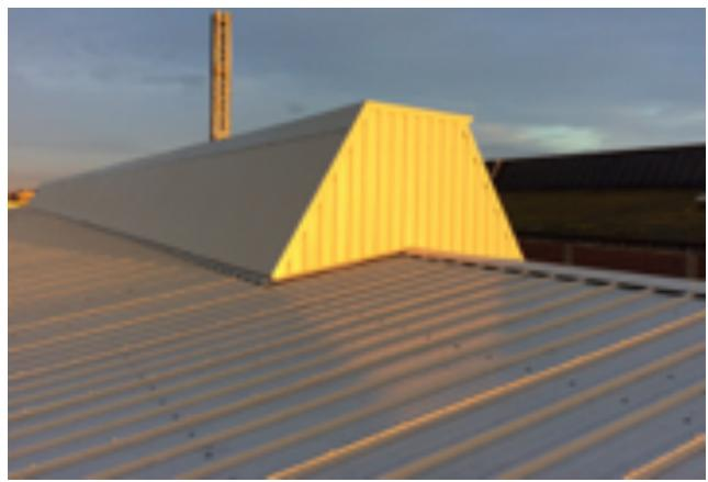
**Far left**: Existing roof areas were dried off and repaired prior to the new waterproofing system being installed.
