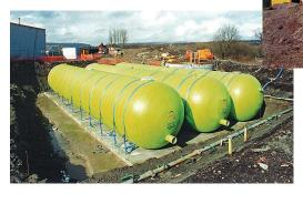
3 x 300 m3 Combined Sewer Overflow attenuator tanks – Dwr Cymru/Welsh Water – Nelson, South Wales
