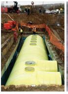
4000 litre/sec. Camplas Bypass 'Filterceptor' taking the entire flow from the giant Ford Engine Plant with (inset) the Camplas 'Divertaflow' valve which can shut off the flow automatically.
