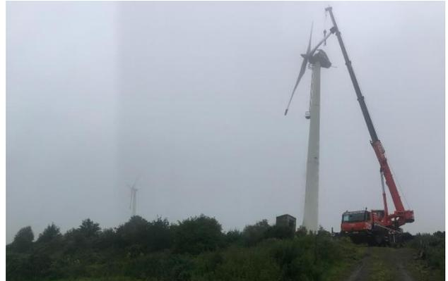
Following final testing at the repair facility, the generator was returned to site, reinstalled and recommissioned. The turbine was then re-energised and the necessary function tests were carried out. On completion, the turbine was fully operational, and the turbine is now maintained by Realise Energy Services under a Standard contract and has continued to run well since the major repair.
