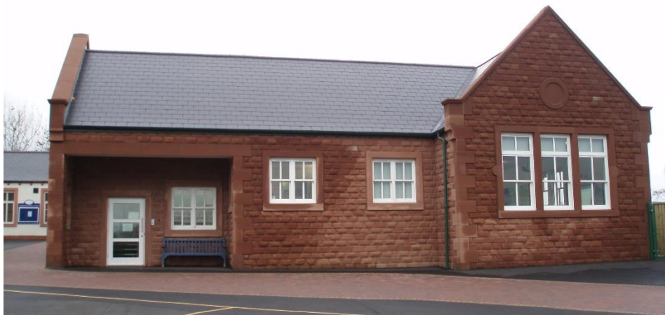
Corsehill walling and surrounds used on a primary school extension
