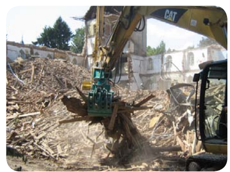
Appropriate for demolition works
