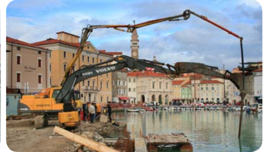
Underwater concreting - Arm extension enables concreting in a higher water depths (longer distance). It guides the funnel to required depth and enables underwater concreting.
