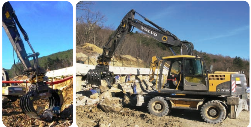
Hydraulic grab BG16 is also appropriate for works of stone laying - making the scarps.
