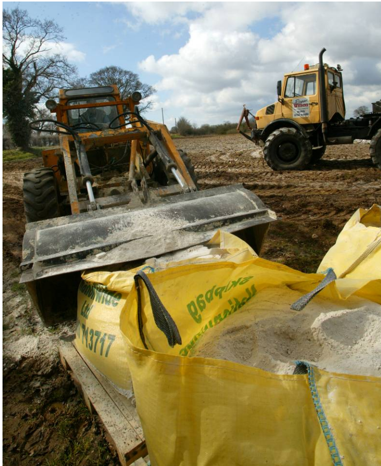
Figure 2 Recycled gypsum supplied in bulk bags
